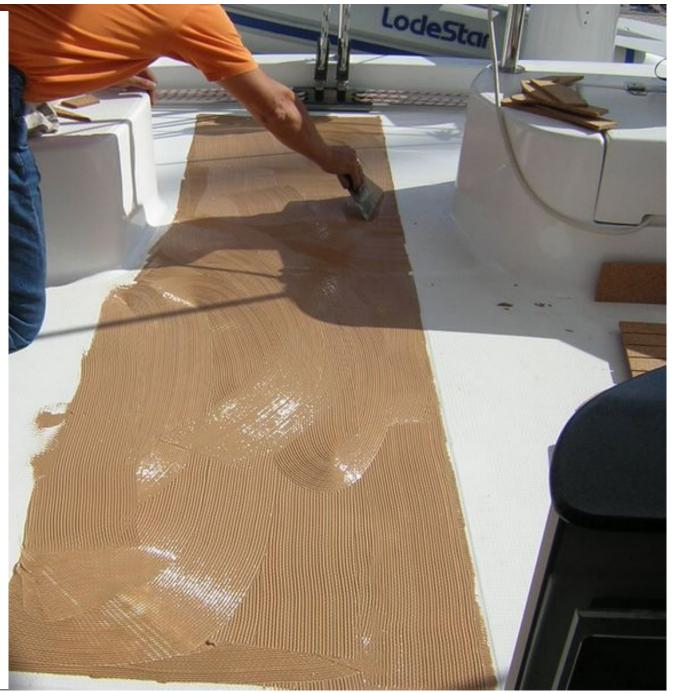
Be sure the adhesive is uniform. Set the first sheet into place on the adhesive. Starting from the center apply pressure working to the outside. Using a rubber mallet and a block of wood will assist. The purpose is to remove any air that may be trapped, setting the sheet well into the glue.
