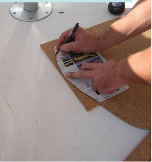
After tracing, cut pieces in two or three passes keeping the blade perpendicular to the cutting surface. Sand the cut edge using 60 grit paper with a sanding block to smooth and shape your cut edge.
