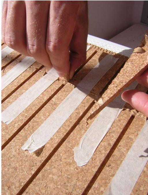
Once all the pieces have been glued we can trace the border pieces. Using a board and the cut border pieces, Position your pieces and trace them onto the sheet for cutting. Now is the time to locate and consider caulking joint seams in relative position to one another.
