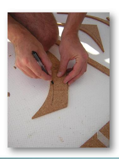
Once the first cut is made, trace a parallel line to the cut edge using a piece of cork of border dimension to ensure the accuracy of the piece.
